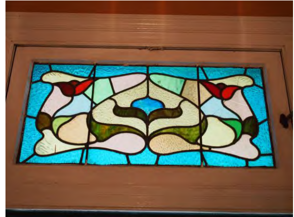
Figure 74. Detail of the leadlight highlight above the front door. This appears to be in very good condition, although some of the glass pieces are slightly cracked, all are original and in position.
