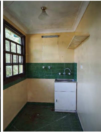
Figures 110-112. A second bathroom and laundry were added as a wing to the rear of the house under a skillion roof, potentially when the deck was added. The windows to these two rooms are timber framed sash but are of uncomfortable proportions and much lighter construction than in the remainder of the house.
