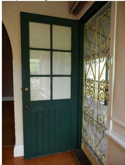
Door to the rear sunroom. This is an external door of similar design to that now on the back door, although the hardware is simpler and it does not include a central handle as is seen on the main doors.
