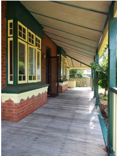
Figures 51-53. The verandahs are deep and sheltering. Floorboards are hardwood and most appear to be original except some replacement where weathered at the outer edges.
