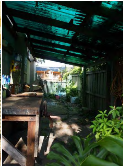
A carport/storage area has been created by adding a skillion roof with green polycarbonate sheet roofing to the space between the garage and the western fence.
