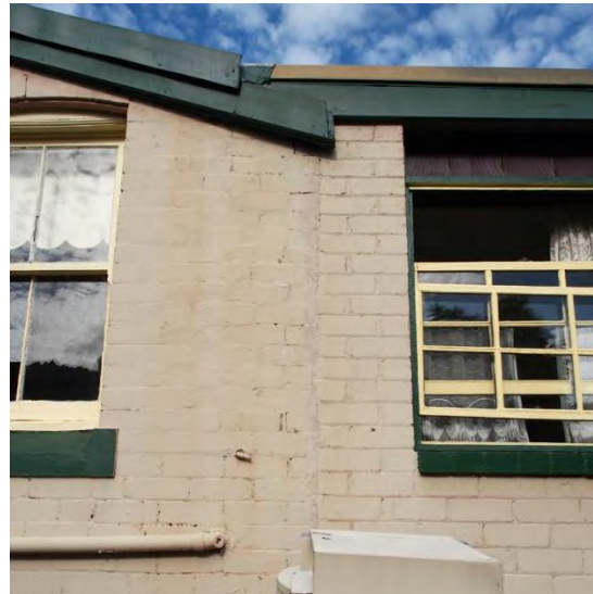
Figure 129. The rear utility wing addition is not built to the same quality as the remainder of the house and elements such as the window sash may need repair.
