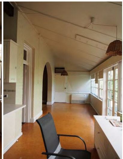
Figures 105-107. The sunroom was created by the enclosure of the back verandah by lightweight glazing. Note the retention of the raked verandah roof line. This alteration was likely to have been made pre-1936 since it is shown as part of the enclosed footprint of the house on the Water Board plans of that year (see Figure 5). The original rake of the roof has been retained and the floorboards covered by cork tiles.
