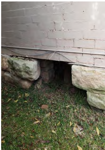
Figures 65-67. Evidence of disturbance to the space now occupied by the bathroom: stonework has been removed to provide access to the subfloor space.
