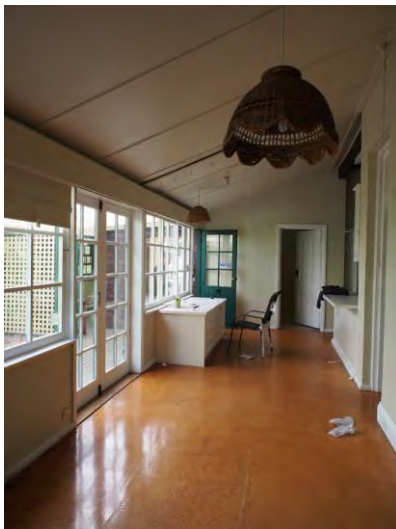
Figures 105-107. The sunroom was created by the enclosure of the back verandah by lightweight glazing. Note the retention of the raked verandah roof line. This alteration was likely to have been made pre-1936 since it is shown as part of the enclosed footprint of the house on the Water Board plans of that year (see Figure 5). The original rake of the roof has been retained and the floorboards covered by cork tiles.
