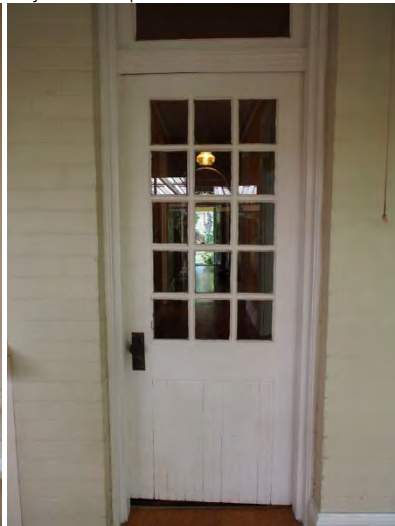
Door to the central hallway. This door was also an external door.
