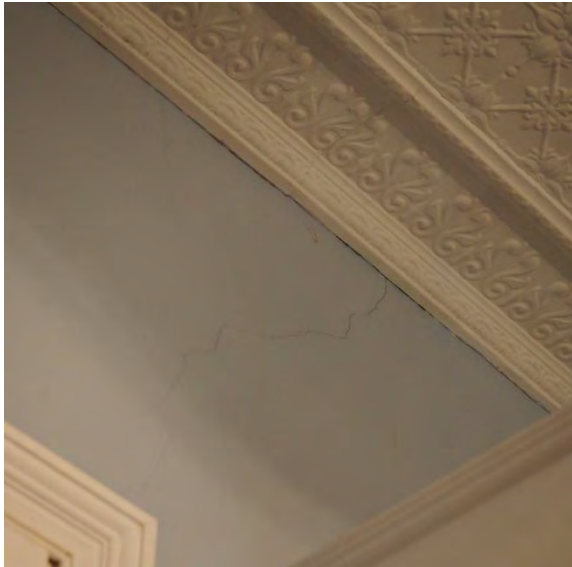
Figures 124-125. Fine cracks to bedroom 3 above door. The slight discolouration of the adjacent cornice suggests that this may have been/is due to water penetration. This should be investigated.
