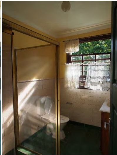
Figures 110-112. A second bathroom and laundry were added as a wing to the rear of the house under a skillion roof, potentially when the deck was added. The windows to these two rooms are timber framed sash but are of uncomfortable proportions and much lighter construction than in the remainder of the house.
