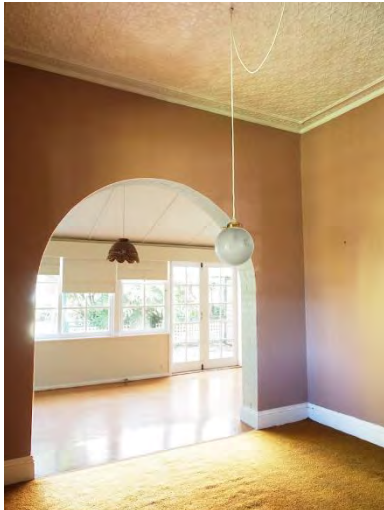
Figures 108-109. Considerable changes have been made to the original rear wall. An arched opening has been formed to the dining room (originally the back bedroom) and the rear wall to the new kitchen has been removed to allow it to integrate with the rear sunroom space. The workmanship of the arched opening reveals that it is not an original detail, although the alteration, which included the partial re-laying of this part of the wall using radius brickwork, has been made relatively neatly. The cutting of the wall to the kitchen space is well concealed by the tiling and cupboards.
